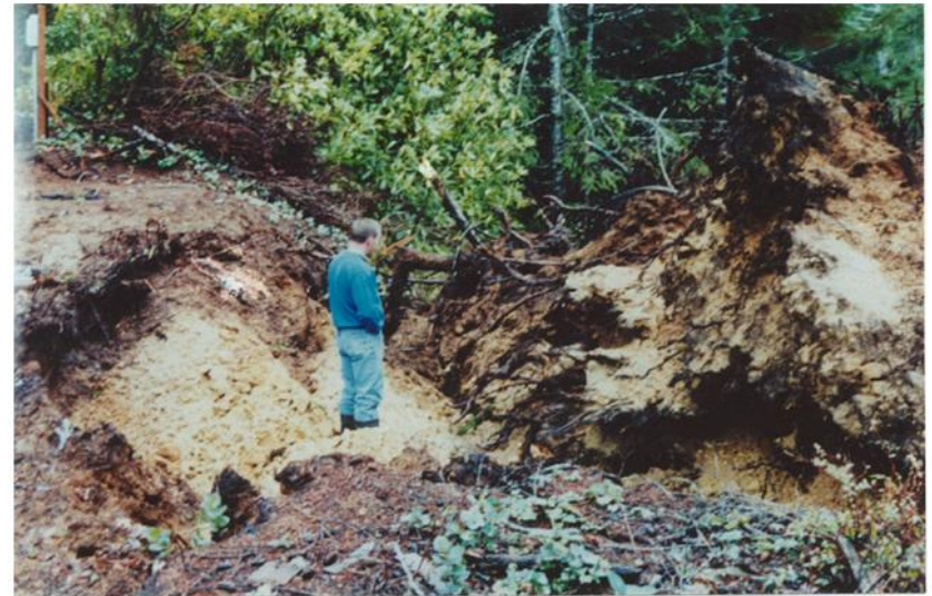
Serious damage by uprooted tree to embankment stability at a dam in Oregon
