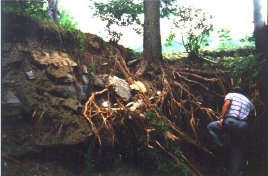
Tree root induced scouring on crest and downstream face of Coffey dam in Kansas
