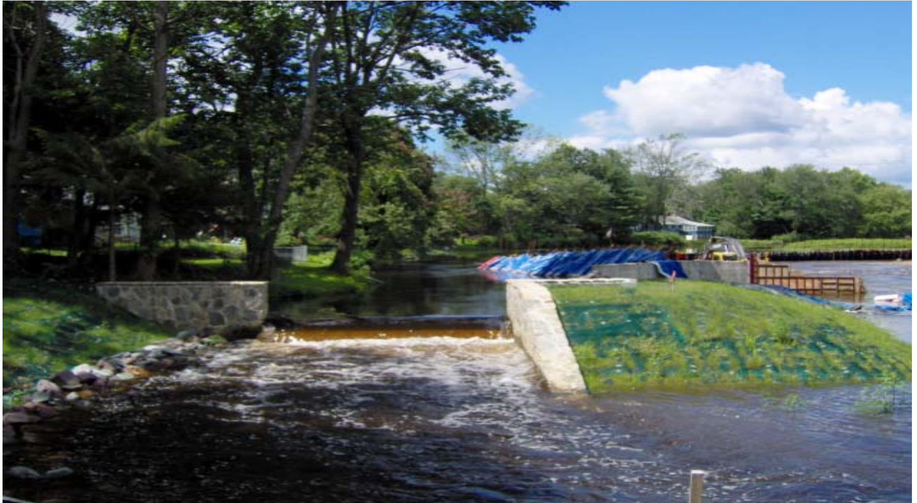
Saturday, Aug. 9, 2008 - Pail Factory Cofferdam Shortly after the breach occurred Auxiliary Dam handles the load
