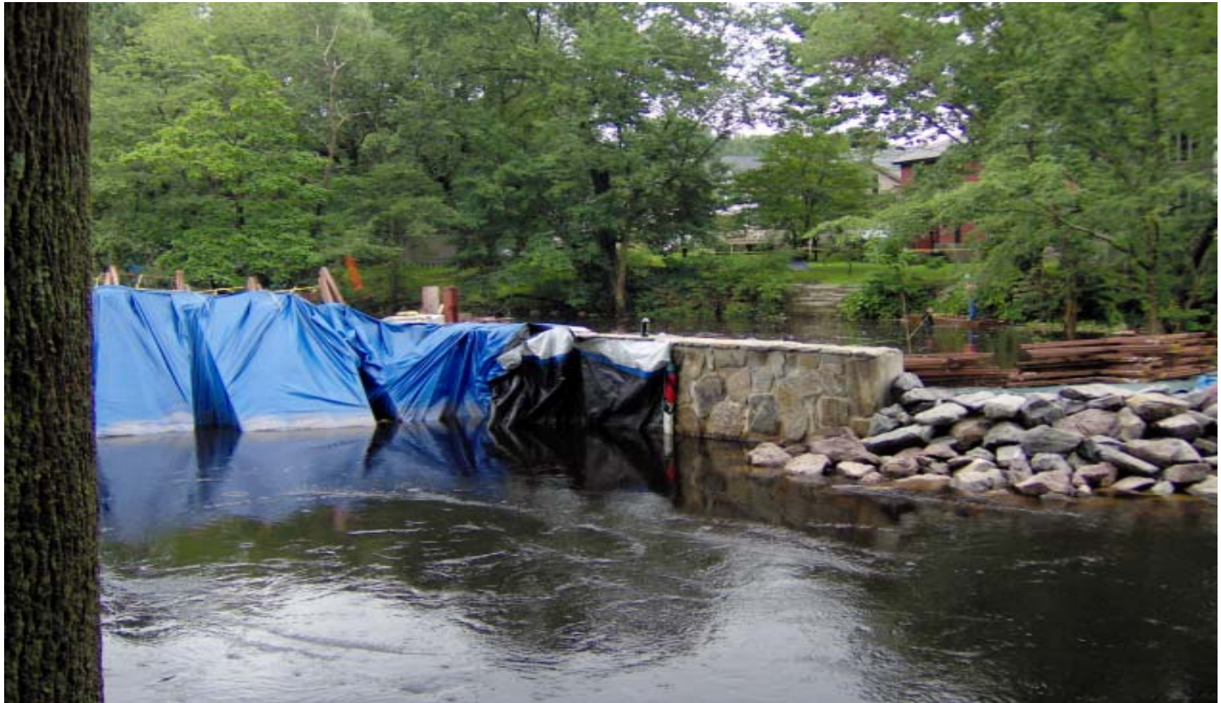
Sunday – Aug. 10, 2008 – Cofferd Dam Breach Water heading toward the Auxiliary Dam
