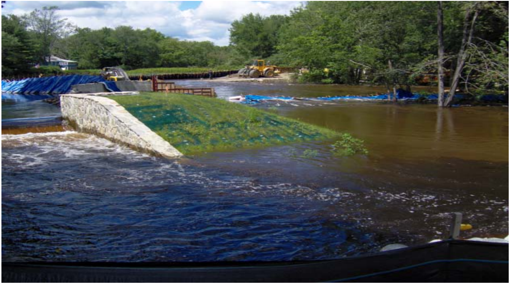
Saturday, Aug. 9, 2008 - Pail Factory Coffe Dam breach at rear left of 1st coffer dam - 2nd coffer dam is down
