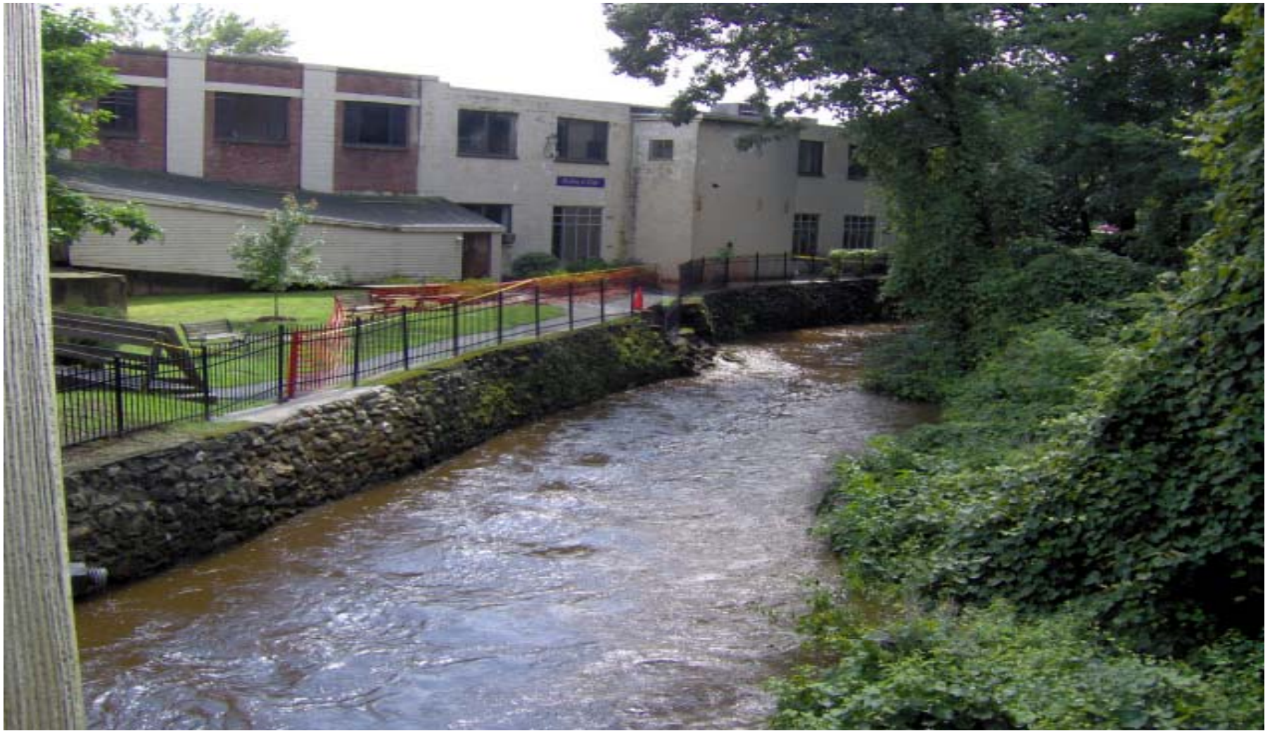
Monday, Aug. 11, 2008 – Nashoba Brook wall damage due to previous weakness in wall and water flow from Pail Factory Cofferdam breach.
