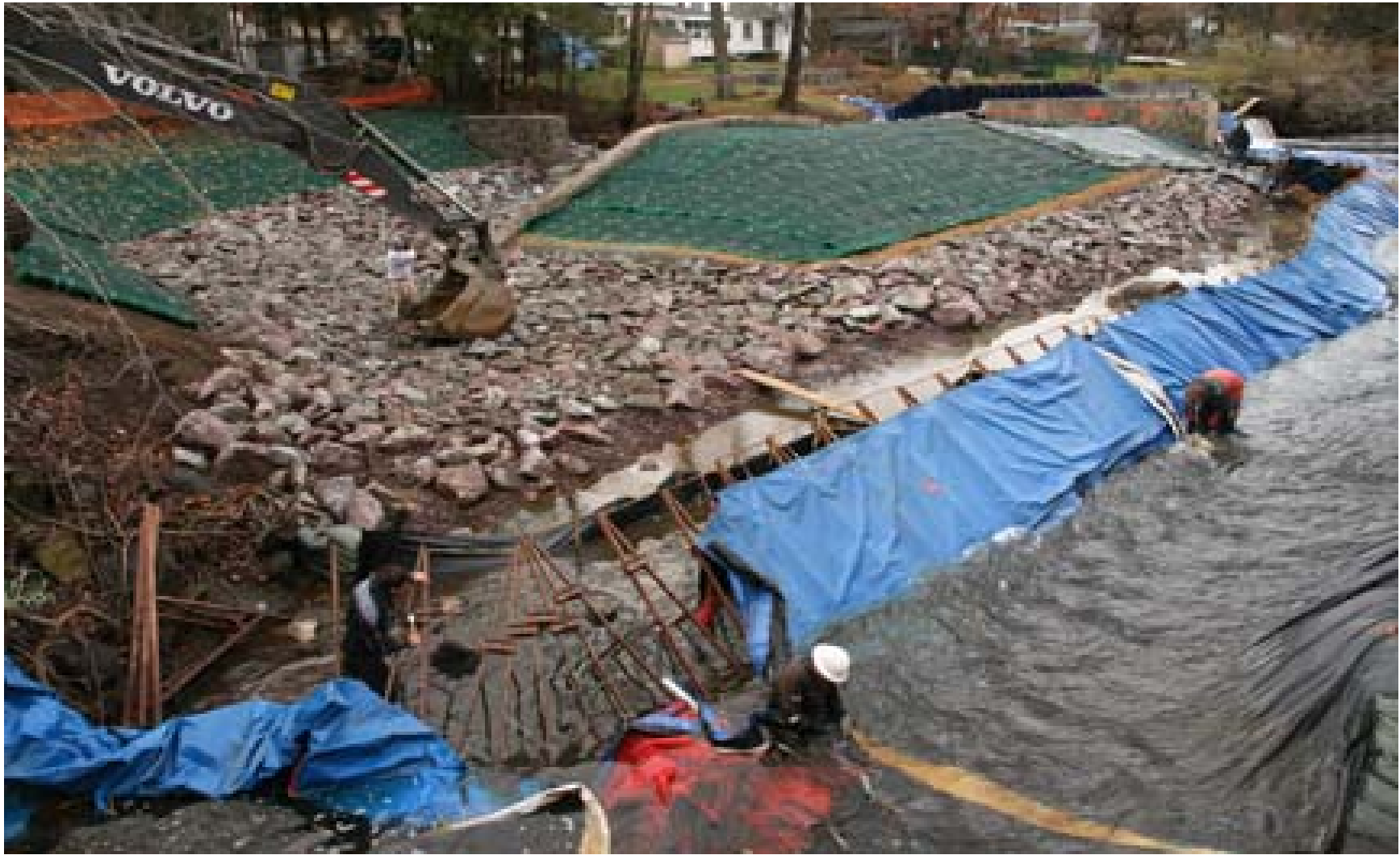
Removing cofferdam and grading new riprap within spillway and along earthworks
