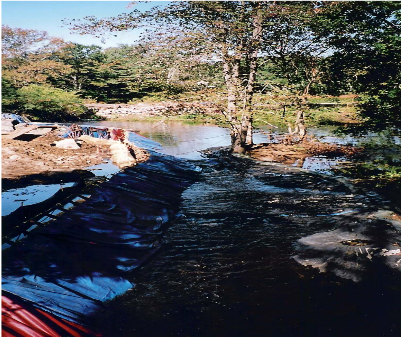
Diversion of water to main stream to begin work on the spillway
