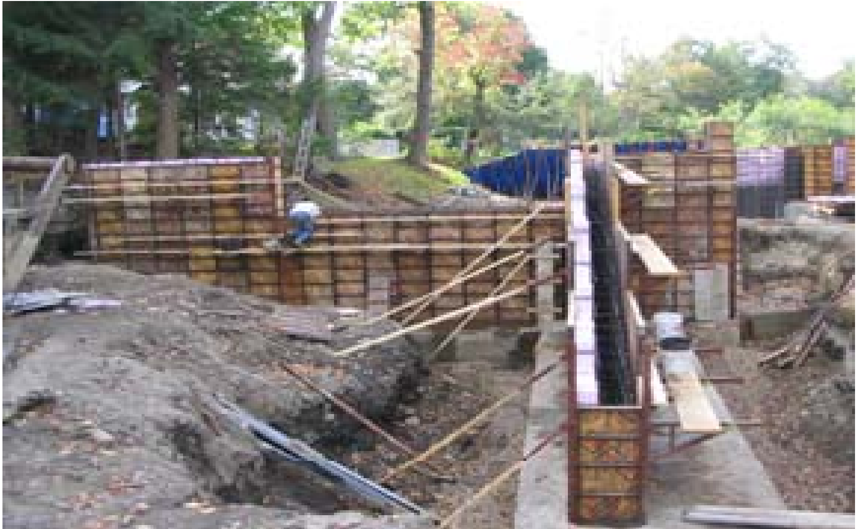
Installation of formwork for new spillway dam and wing walls
