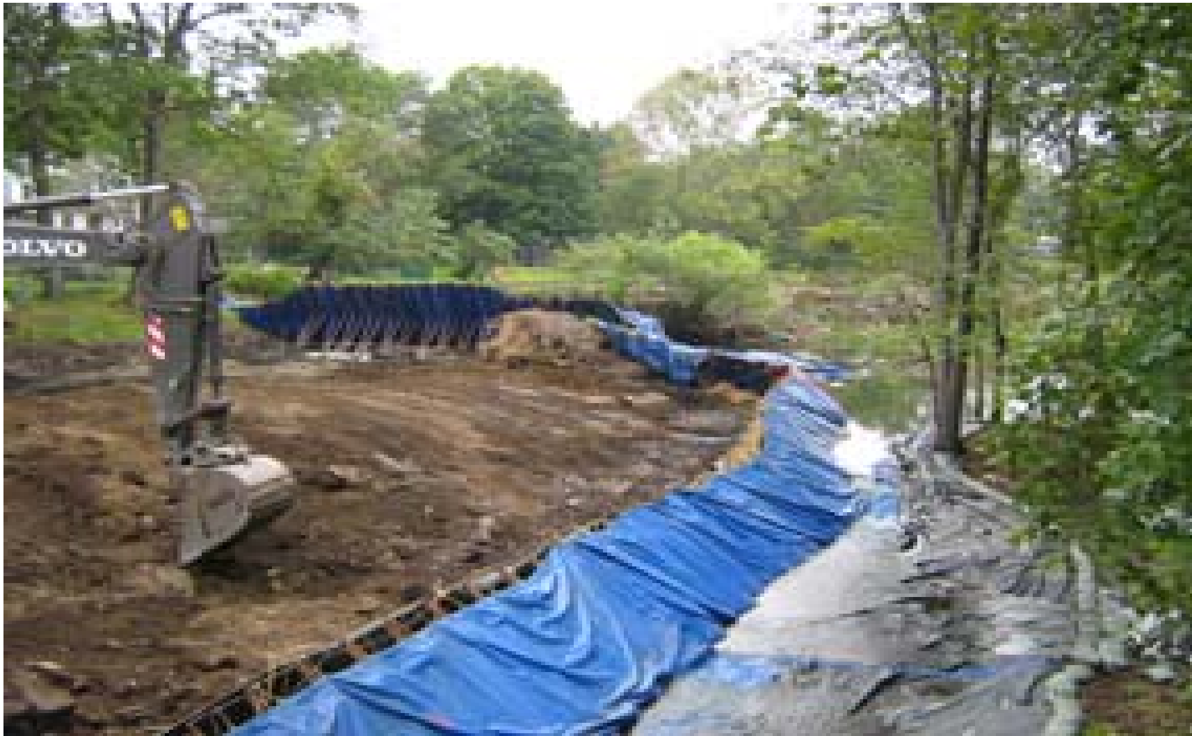
Grading earthworks adjacent to new spillway
