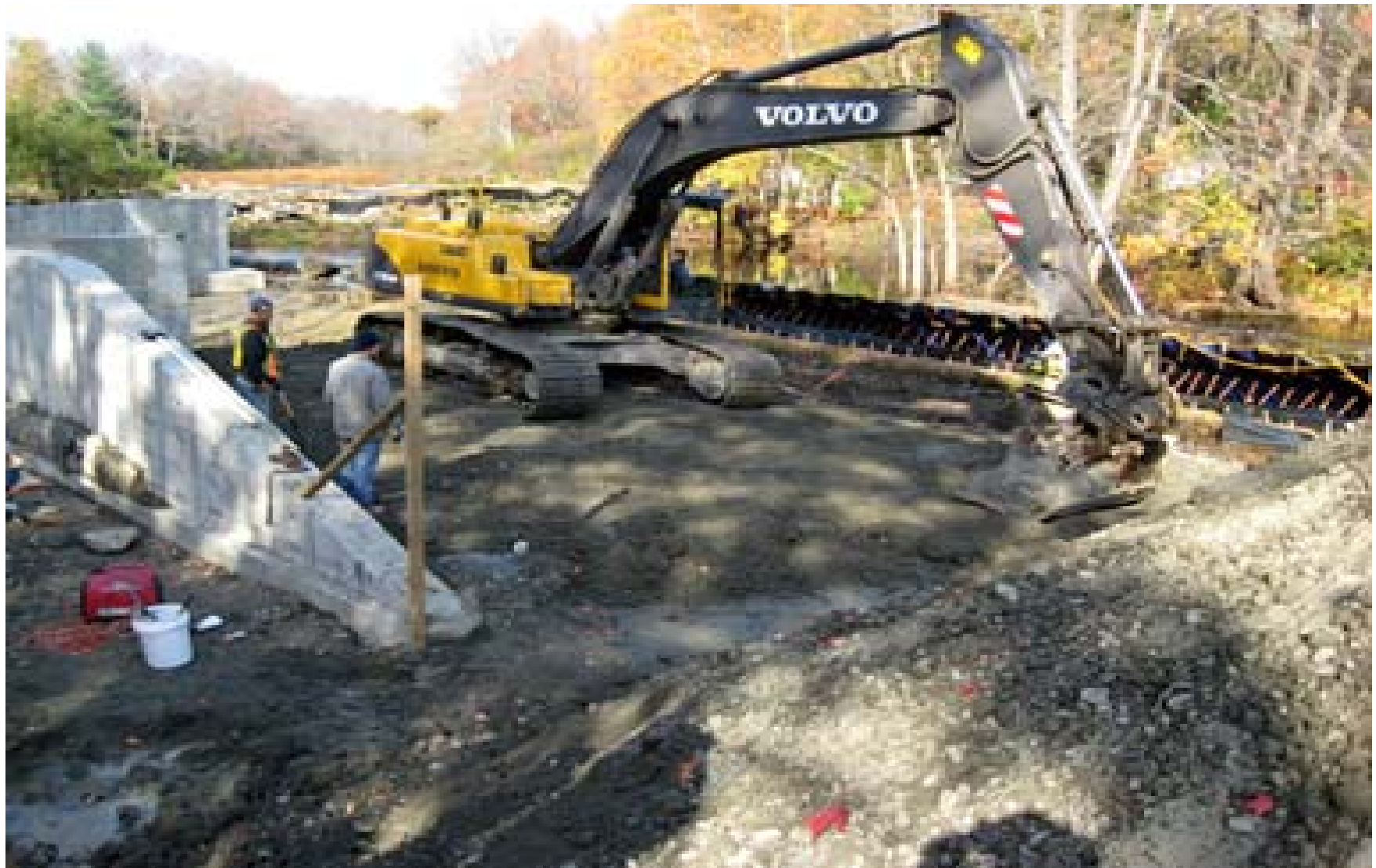
Grading of earthworks adjacent to new spillway, preparing for additional backfill
