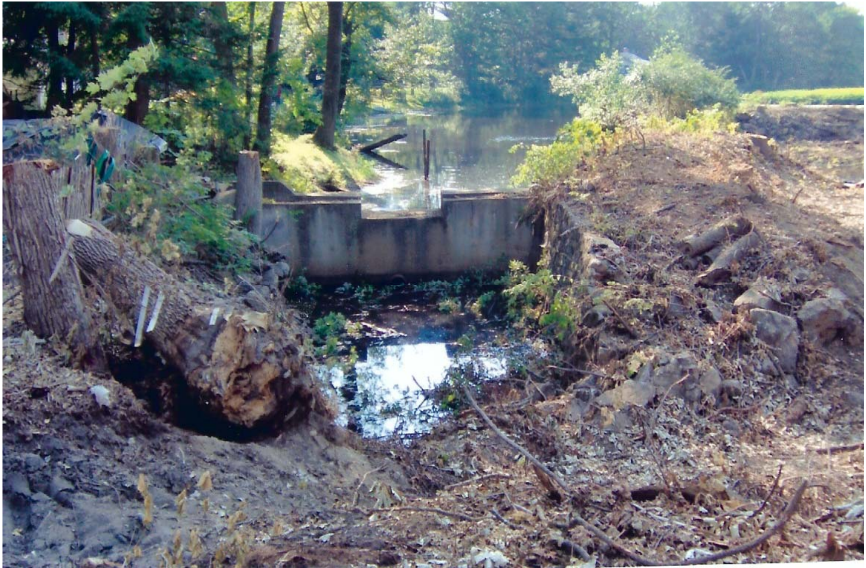
Spillway is cleared in preparation of installation of the Cofferdam
