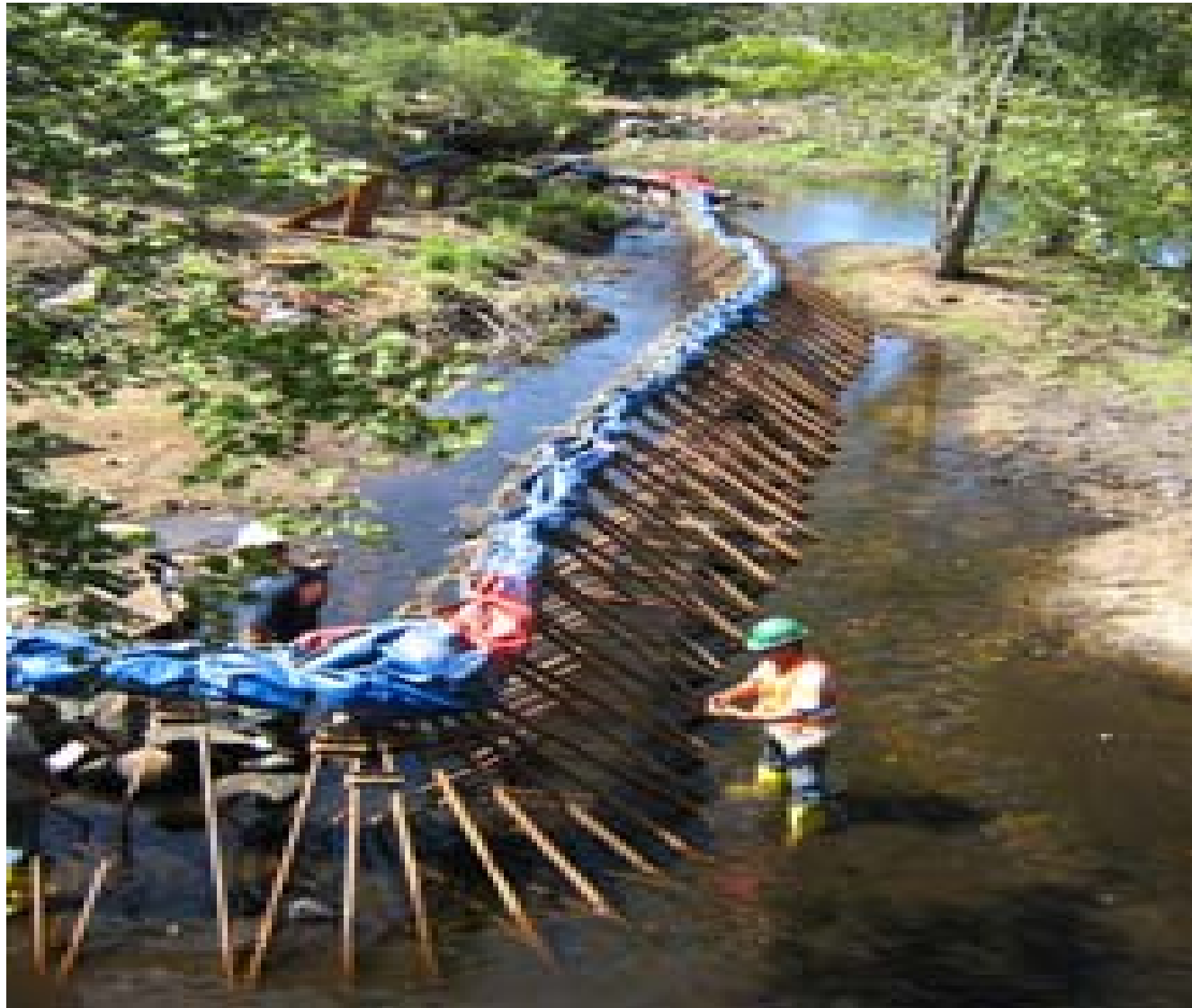
Installation of cofferdam
